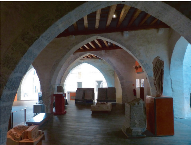
Figure 8 The house of Mestre Peña, now the historical museum, is an example of fourteenth-century modular architecture based on pointed arches.
