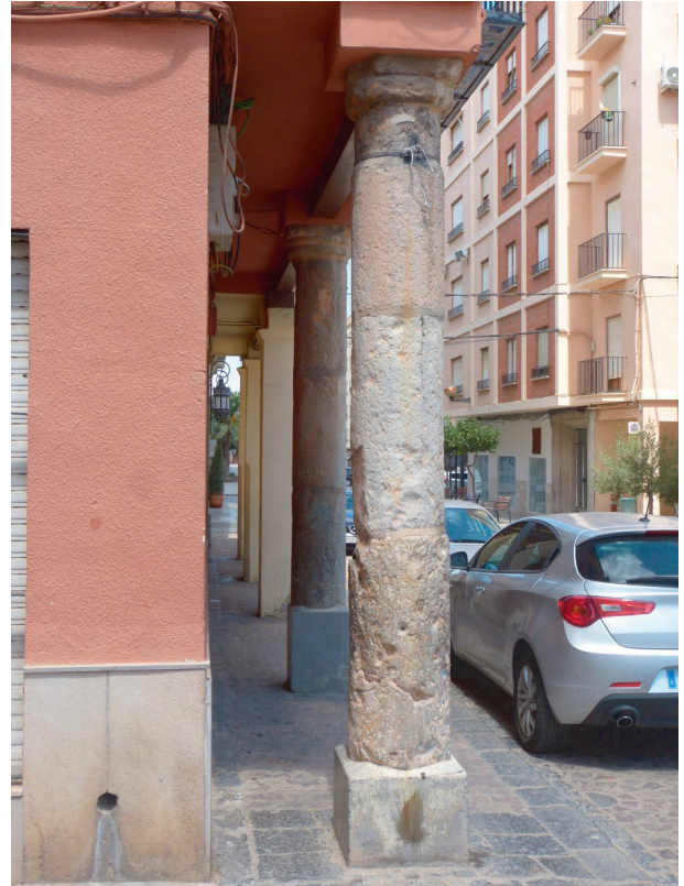
Figure 9 Portico in the Plaça Major reusing a Tuscan column.
