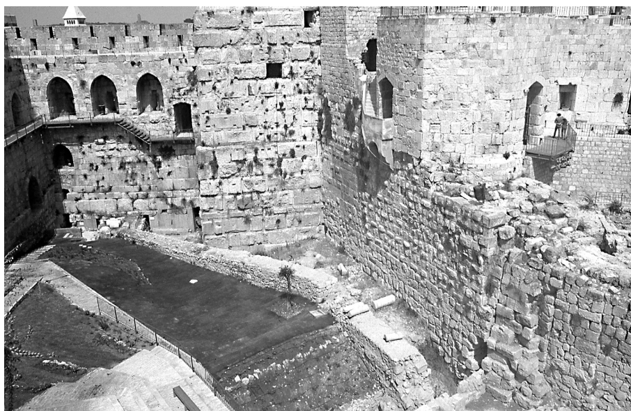
Fig. 6 : The outer side of the Hasmonean-period First Wall in the courtyard of David's Citadel. On the right, section constructed with headers; on the left, section constructed with marginal stones and central protruding boss.
