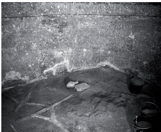
Fig. 4 : Photo of interior of cistern in 1997, showing raised lumps in floor, jug in situ in Mound B, water line at top and repair line.
