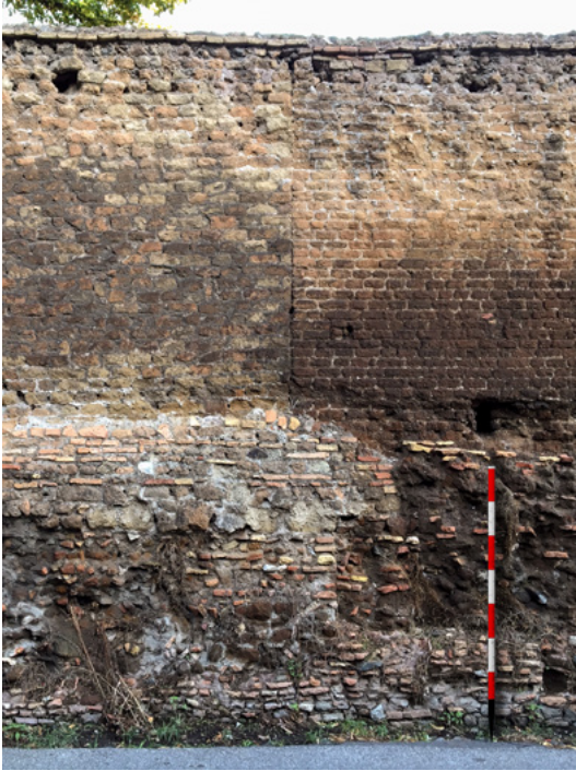
Figure 3. South-east frontage (PR2) - detail: connection between the walls in small blocks (right) and the earlier structure in roughly refined rubble (left).
