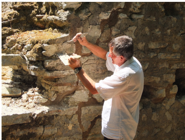
Figure 3. Shëndëlli workman repairing a Venetian wall at Butrint (photograph by D. Phelps).
